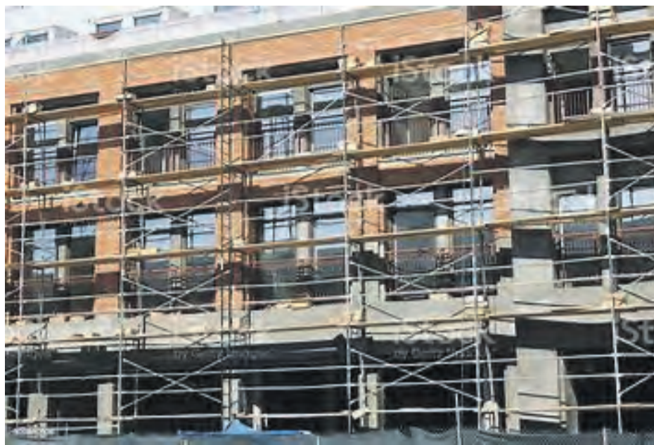
A building under construction.
